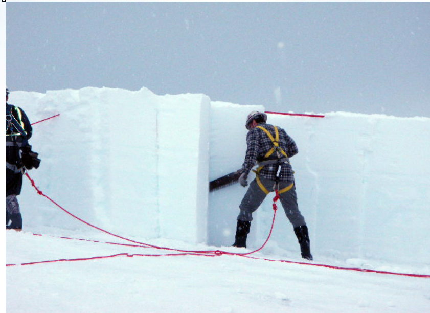
Tank top snow removal
