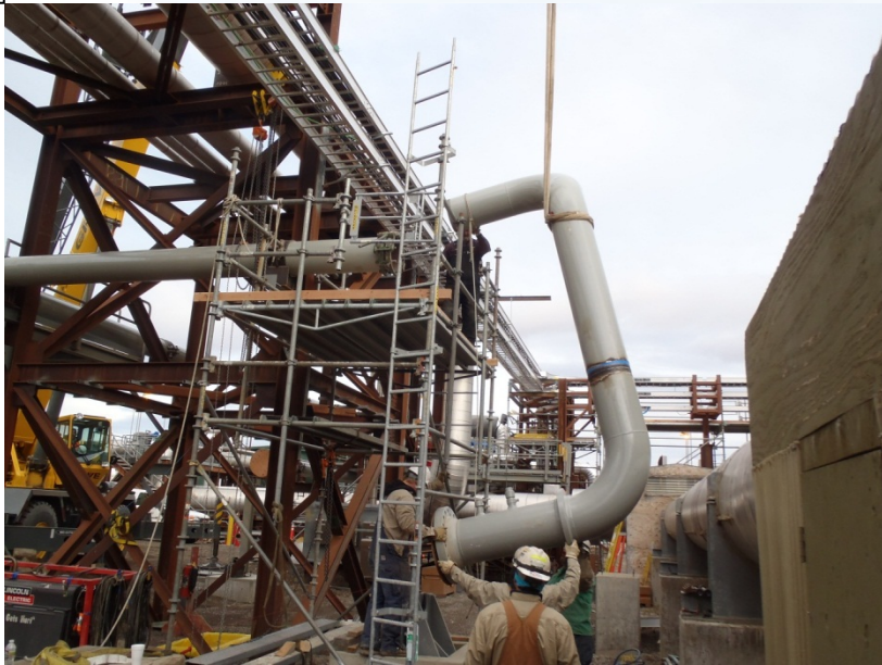
Recirculation at a pump station adds 7-10. Winter recirculation at PS 3, 4, 7, 9.
