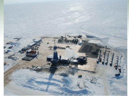
ExxonMobil will be the operator of the Point Thomson field east of Prudhoe Bay.
