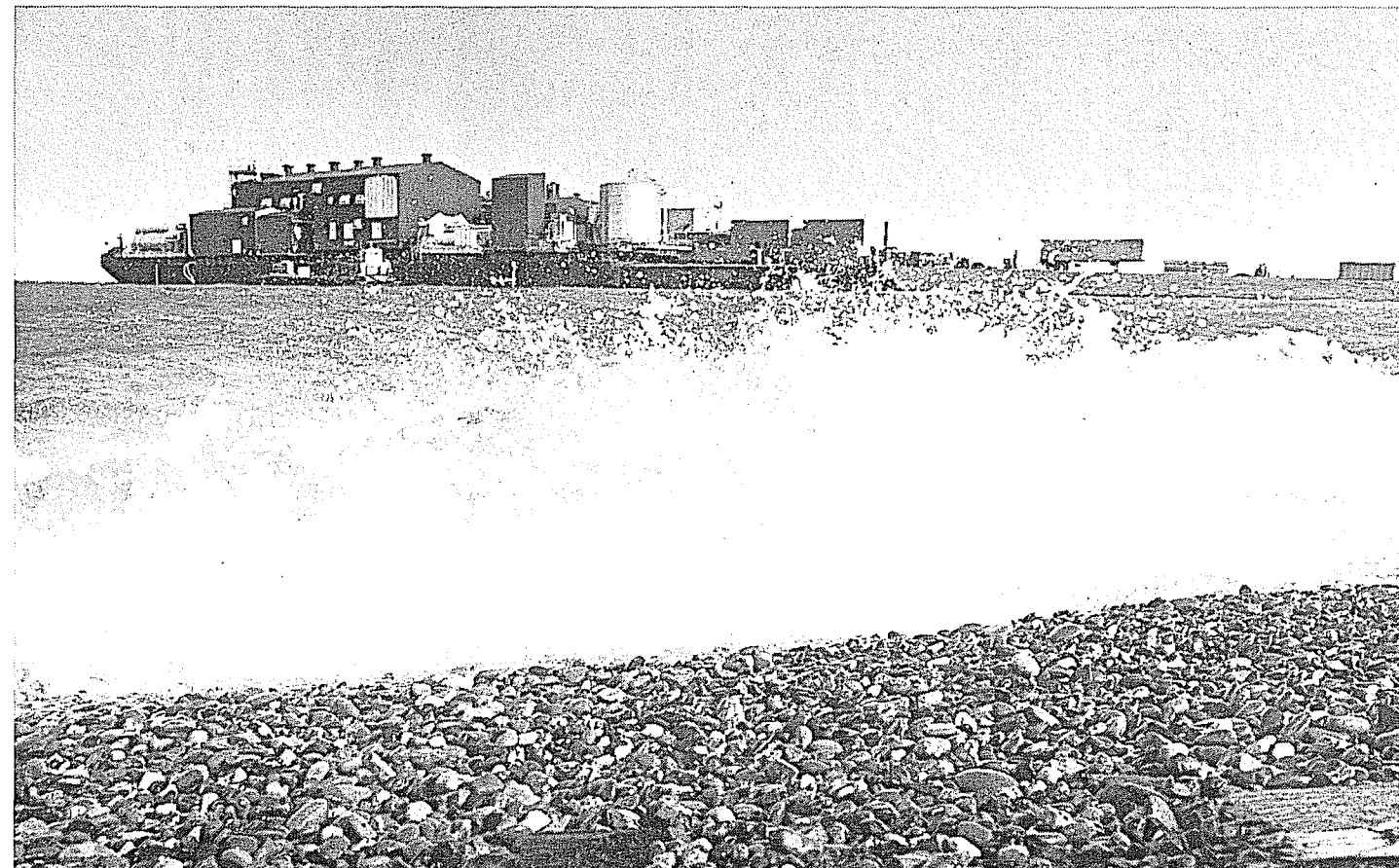
The construction of North Slope production facilities, including these giant modules, funneled millions of dollars into the national economy. These modules were transported by barge to the North Slope.
