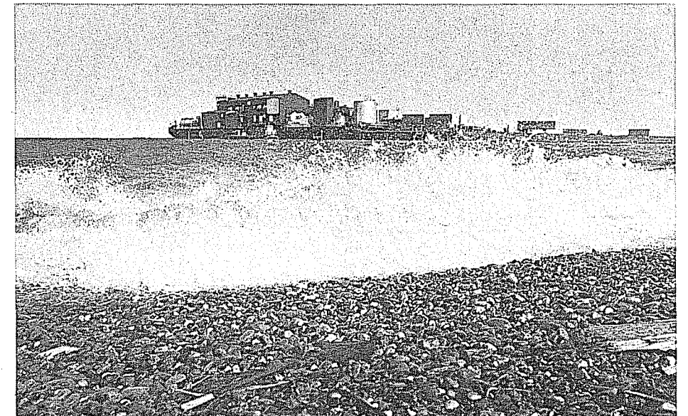
1986 will bring the biggest summer sealift ever and the largest construction year yet to the North Slope. Oil companies say such activity is the result of a stable tax climate, adopted by the legislature in 1981.
