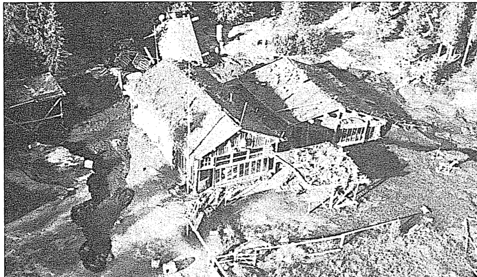
Over a foot of silt covers the floors of Doug Vaden's cabins on North Fork Island after three years of flooding. Toni Hankins, Vaden's granddaughter, said the damage could have been avoided with a few hours of work upstream on a gravel bar of the White River. The National Park Service would not permit the work which Hankins said would have returned the river into its original channel while saving the island from destruction.
