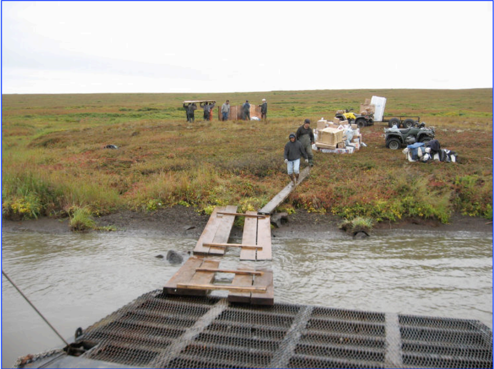
Taking the housing packages off the barge
